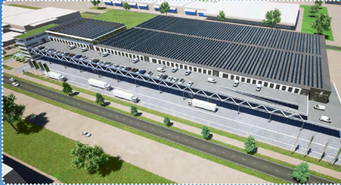
Parking above dock
