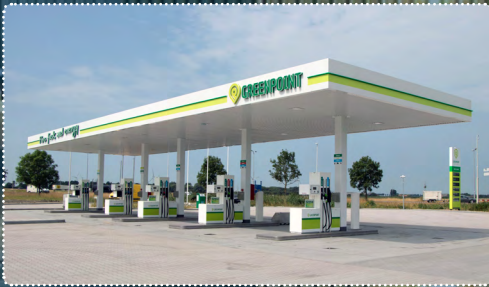
Clean energy hub Van Kessel
