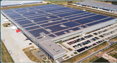
Rhesus solar panels
